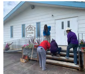
Prepping to paint church steps
